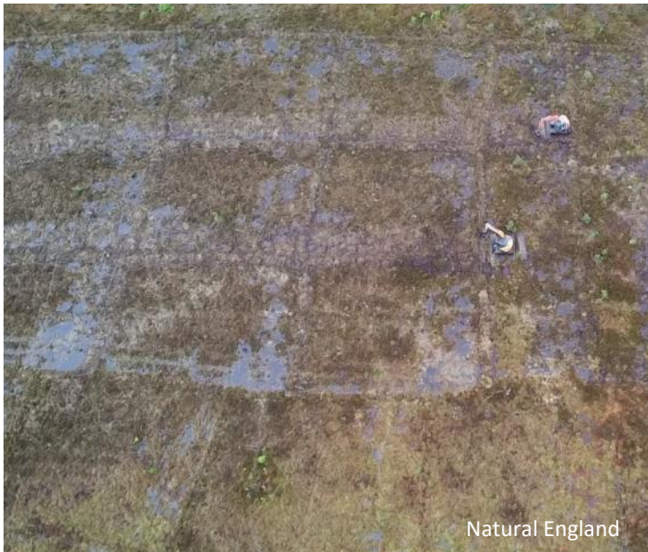
Above: Peat bunding being carried out on the Duddon Mosses. The grid-like structure is designed to hold water on the bog for as long as possible.
