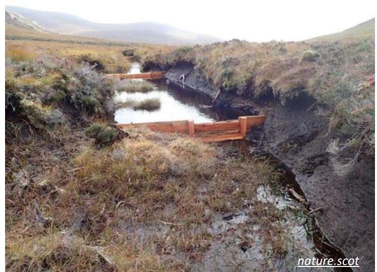
Below: Wooden bunds installed in a degrade peatland to hold back water.
