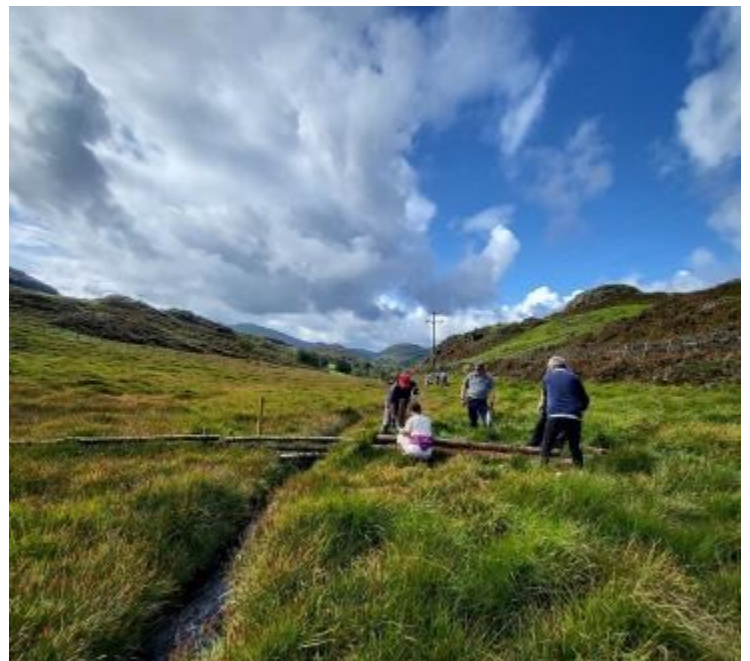
Volunteers build a leaky dam extension
