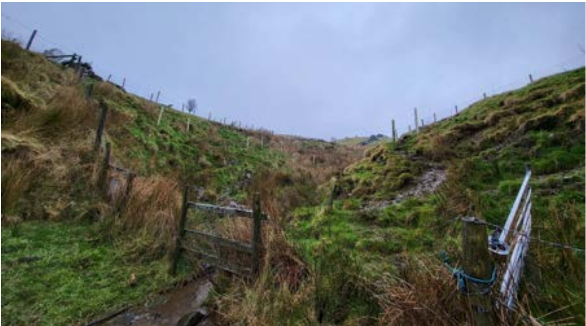
Figure 16: Recent fencing and tree planting upstream at Standish Cote.
