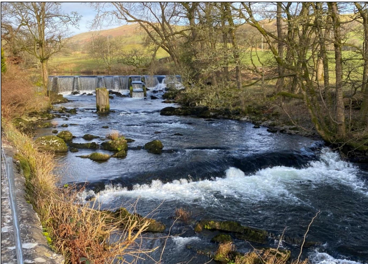
Figure 3. View from right bank looking upstream towards Bowston Weir, showing section rock ramp is to be located
