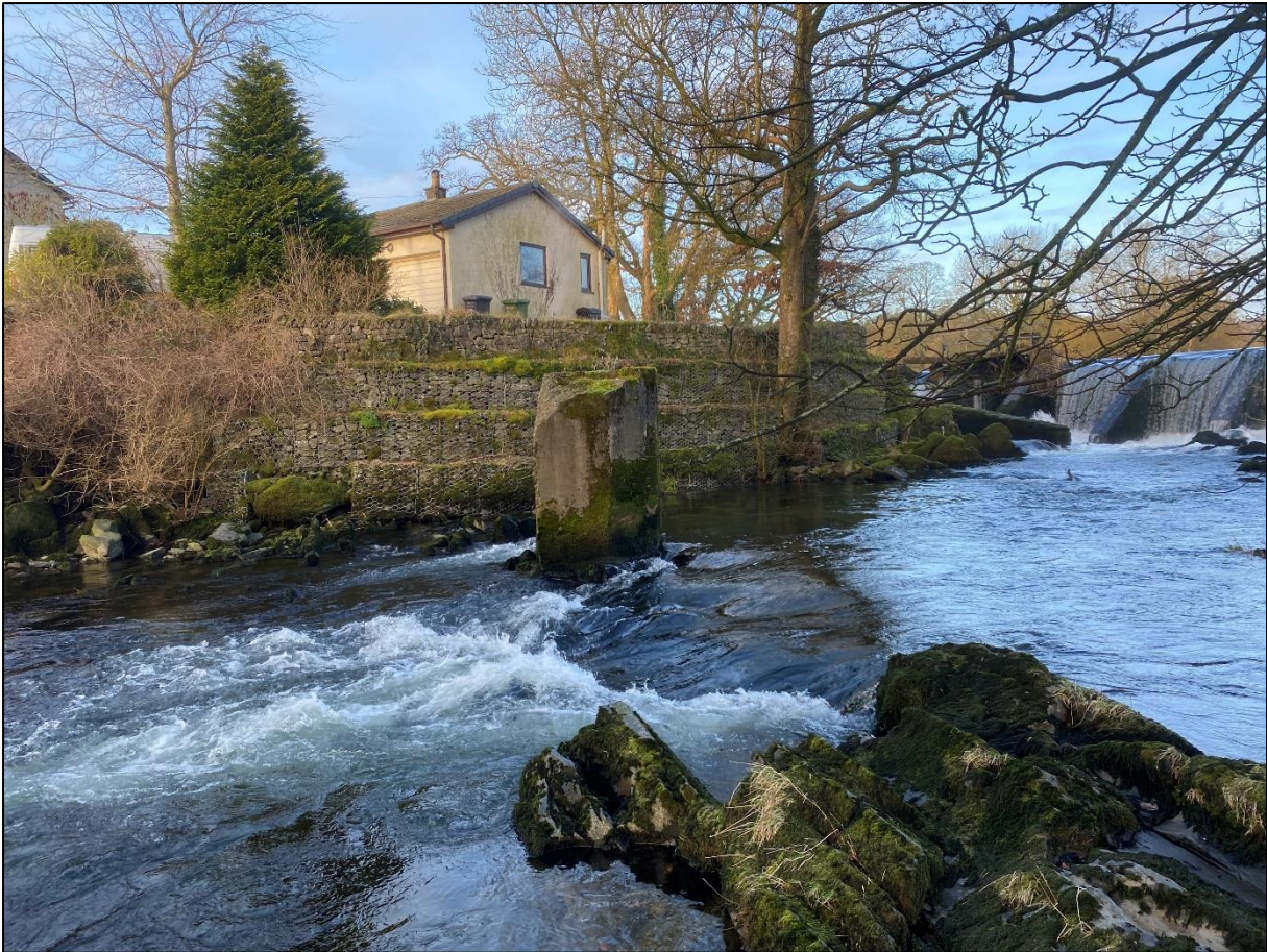
Figure 4. View from left bank downstream of the weir, indicating concrete pillar to be removed
