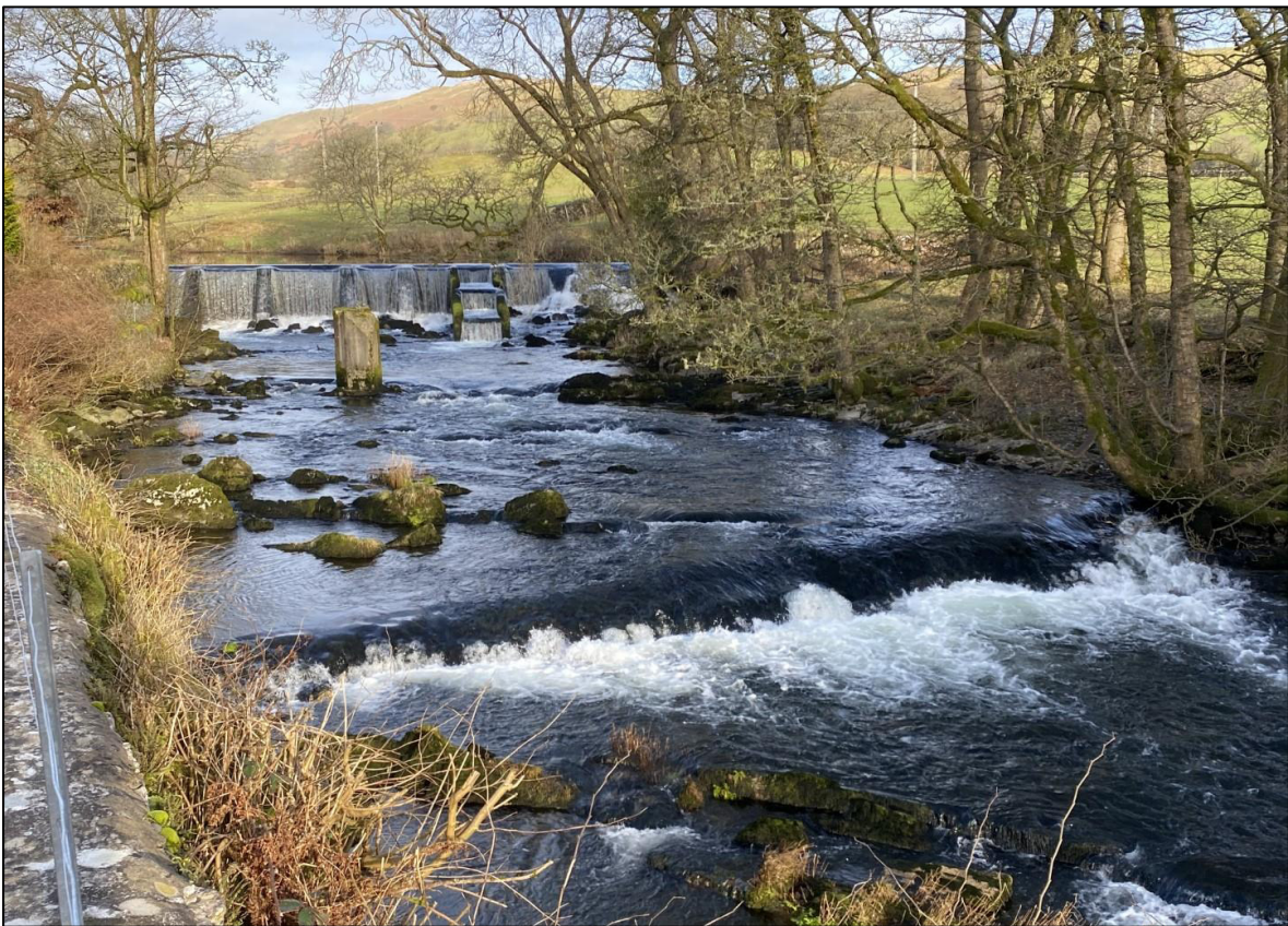
Figure 2.3. View from right bank looking upstream towards Bowston Weir, showing section rock ramp is to be located.
